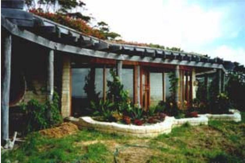
Close up exterior view of Brown House - earth covered roof, indoor-outdoor gardens and ponds, load bearing earth walls, passive solar design, composting toilet.
