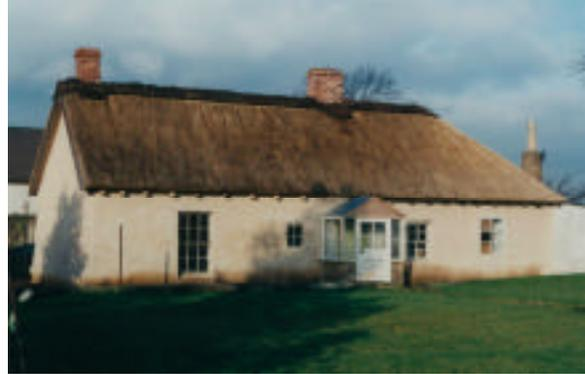
The repair programme involved the reinstatement of the thatched roof, a heather-turf and clay ridge and consolidation of the mudwalls. The main external problems concerned neglect of the building and inappropriate repairs carried out in the recent past. The sequence of works involved removal of cementitious finishes, repair of the earth and the reinstatement of lime coatings once the walls were made good.
