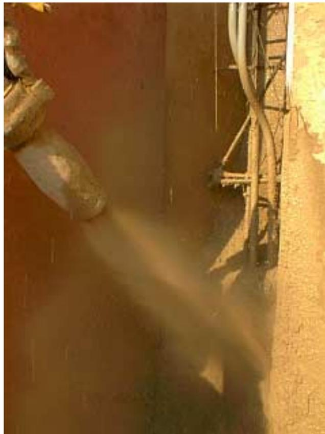
In addition to the increased speed of installation, there are several other factors that make pise' a more practical, efficient, and economically viable method of constructing monolithic earth walls than rammed earth.
