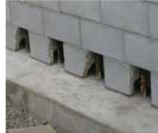
**Figure 5** Basement for house with earth retaining masonry basement – close-ups of reinforcing and cleanout cells.
