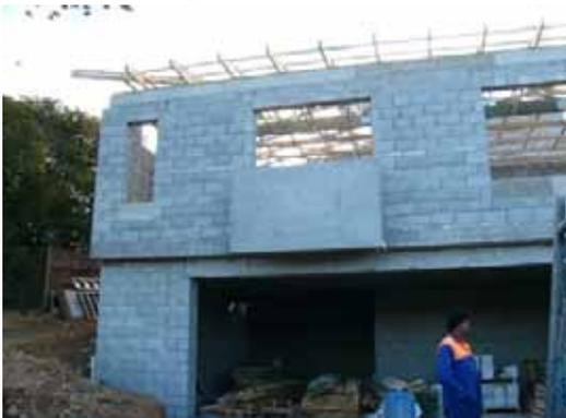
This second example in figure 6 is another large masonry house showing the concrete bond beams at floor and roof levels.
