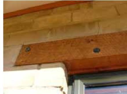
**Figure 8** Pressed Earth Brick House with close view of lintel detail
