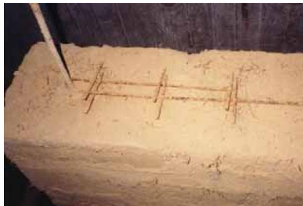
**Figure 20** Reinforcement detail - vertical rods in holes through the adobes and horizontal reinforcement wrapped around the vertical rods, now geogrid is more typical for horizontal reinforcement
