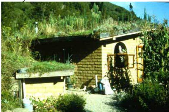
Adobe bricks sometimes use straw or a cement stabiliser which is also used in mortar in the walls.
