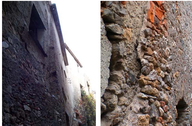
Figure 2: Spurs (on the left) and wall thickenings (on the right).
