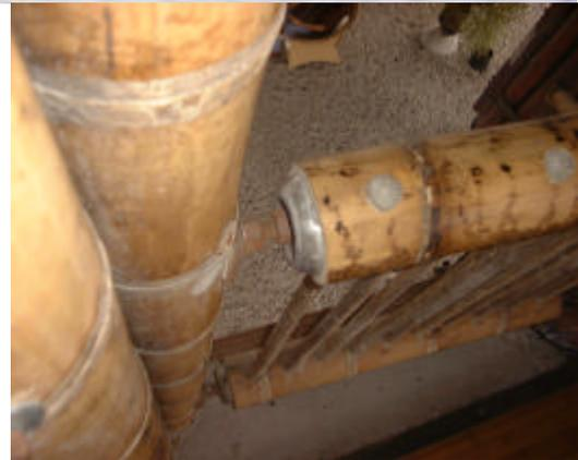
*Almost nobody noticed the deft use of recycled coke bottles that keep the mortar from coming out the ends of the handrails. Filled with mortar, the clear plastic looks like stone.*
