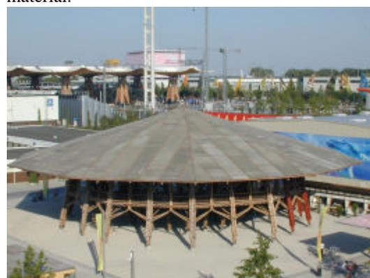
*The surprising innovation of a bamboo-cement composite roof board ([www.taiheiyu-cement.co.jp](http://www.taiheiyu-cement.co.jp))*
