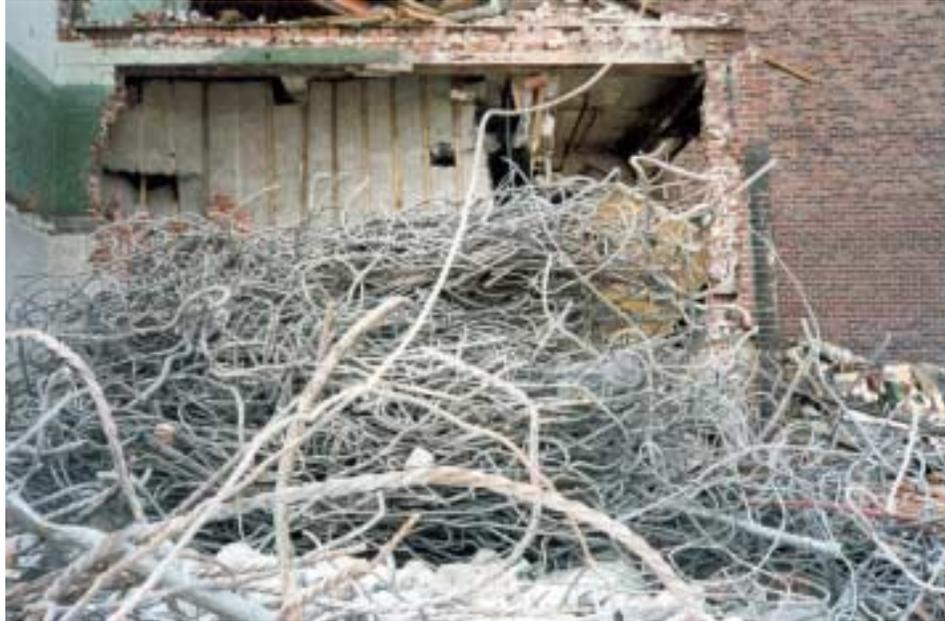
**Figure 5: Concrete Reinforcement at Demolition Site Separated for Recycling**
